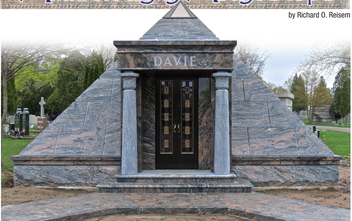
The construction of the Egyptian pyramid mausoleum in Range 7 was completed on May 3, 2019. Photo by Richard Reisem.
