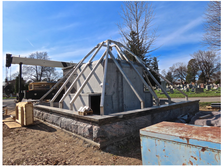
Unlike the pyramids of Giza, here, steel framework holds the 3-inch-thick blocks of granite. Photo by Richard Reisem.
