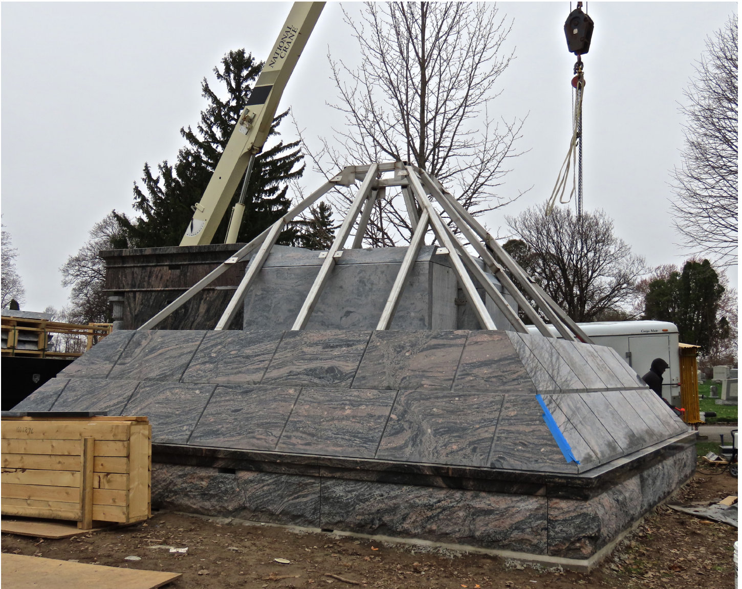
Although the granite was scored to look like rectangular blocks, the stone was delivered in large slabs in order to maintain the flowing rainbow lines in the granite. Photo by Richard Reisem.
