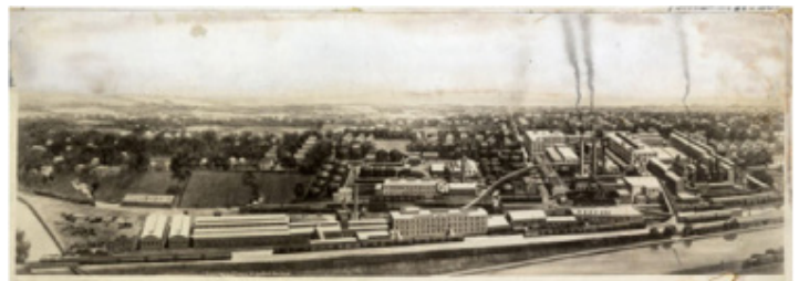
The Socony Vacuum Oil Company in 1925. Photo courtesy ExxonMobil.
